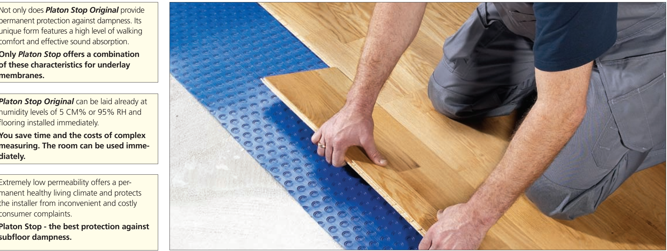
1. Concrete slab 2. Platon Stop Original 3. Parquet or laminate flooring
