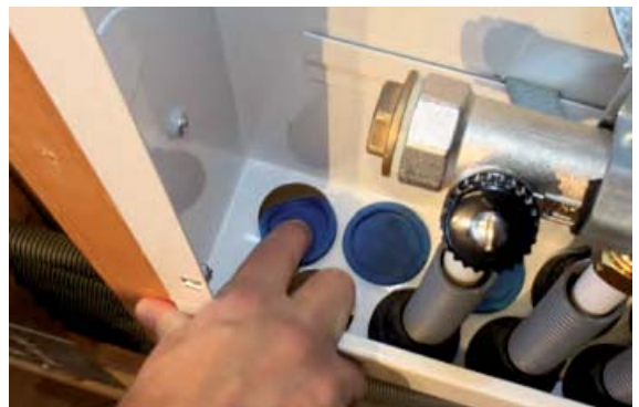
10. The required number of blue rubber plugs are inserted in the holes which are not fitted with the cabinet pipe inlets (these are supplied as standard with the cabinet).
