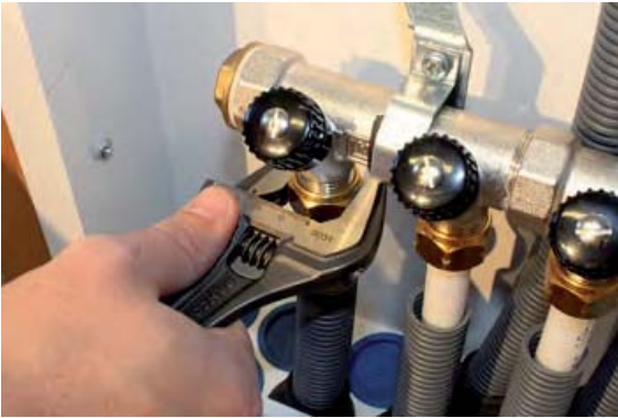
11. Connect the pipes to the manifold.
