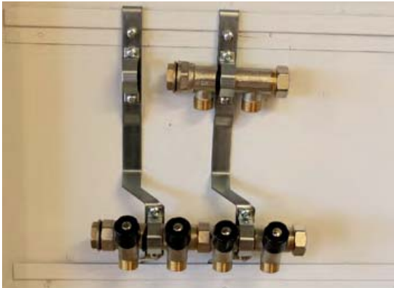
6. Complete assembly of the manifold in the bracket.
