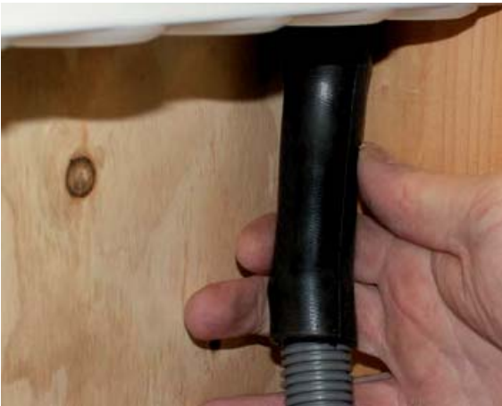
12. The supplied rubber sleeve is slipped onto the outlet for leakage indication. The conduit which is used for leakage indication is inserted into the rubber sleeve. The maximum recommended conduit length is 1.5m and is laid with a slope against the drainage (see Item 2).
