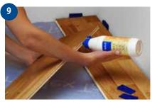
Boards with Tongue & Groove should be point bonded. That is a generous line of glue, about 10 cm long, placed in the groove with a halfmeter intervals. The groove in the short end should be glued all the way.
