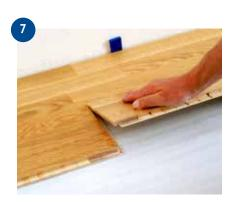
Fold the panel down in a single action movement with a slight press to the short end of the previous panel. During the fold down, make sure the panels are tight against each other.
