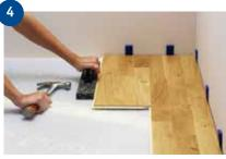
Start the second row with the rest of the cut board. Ensure that all the short end joins are staggered from the short end joins of the other row by at least 50 cm for boards longer than 1250 and at least 30 cm for boards shorter or equal to 1250 (e.g. Viva).
