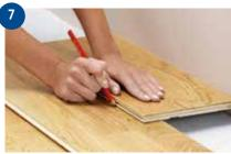
Final row: When you get to the final row, it is possible that the boards will not fit width wise. In this case, place the final board with the tongue facing the wall, on top of and edge to edge with the lastbut-one board. Place a spare bit of board on top and measure the gap by running the bit of board along the wall and marking with a pencil where to cut the final board.
