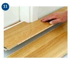
Then tap the board sidewards with a pull bar. Finish by placing spacers in the expansion gap between floor and wall. Now that the floor has been installed, skirtings and any joining strips can be fitted but don't forget to remove all the spacers.
