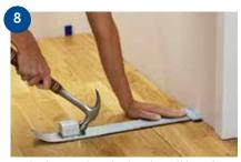
Tap in the sawn board using the pull bar. If the final row of boards has not been cut, the tongue must be sawn off in order to keep an expansion gap. If installing T & G place spacers along the final row of boards too. Now that the floor has been installed, skirtings and any joining strips can be fitted but don't forget to remove all the spacers.
