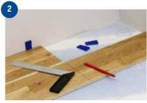
At the end of the row, turn the last board so that it lies tongue to tongue. Push the short end tightly against the wall. Mark where to cut with a pencil 8-10 mm from the previous board's short end to give you an expansion gap when the board is tapped into place.
