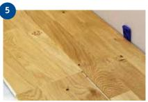
Viva Ultraloc, which has a middle layer of HDF, is tapped together along the long side first. Then tap the short ends together. For other Ultraloc boards the short ends are tapped together first, followed by the long side, starting with the free end. The long side groove must be placed against the tongue for this.
