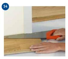
Doorframes can be removed and moved up, but it is usually easier to saw them off. Use a loose floorboard as a height template and saw the frame with a fine-toothed saw. Push the floor under the frame. Ensure that the floor is not wedged between the subfloor and the frame.
