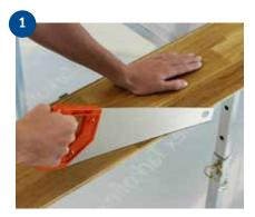
Before installing the first row, the part of the groove profile which sticks out must be cut off.
