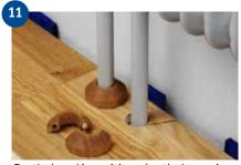
Tap the board in position, glue the loose piece in place, fit a spacer against the wall and cover with pipe collars.
