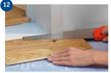
Doorframes can be removed and moved up, but it is usually easier to saw them off. Use a loose floorboard as a height template and saw the frame with a fine-toothed saw. Push the floor under the frame. Ensure that the floor is not wedged between the subfloor and the frame.
