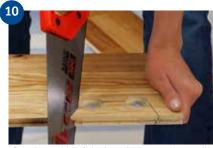
If the long side of the board meets a pipe: Drill a hole with a diameter min. 16 mm greater than the pipe diameter to give an expansion gap around the pipe. Mark with a pencil where to saw. Saw off the bit which will fit behind the pipes, closest to the wall. Cut at an angle as shown in the picture. If the pipes are located along the short side of the floor, cut the board at a 90° angle straight through the holes.
