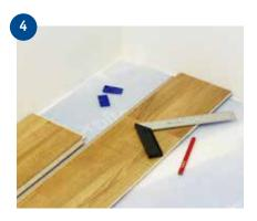
At the end of the row, turn the last board so that it lies tongue to tongue. Push the short end tightly against the wall. Mark where to cut with a pencil 8-10 mm from the previous board's short end to give you an expansion gap when the board is tapped into place.
