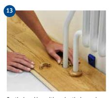
Tap the board in position, glue the loose piece in place, fit a spacer against the wall and cover with pipe collars.
