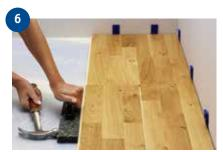
Continue installing the subsequent rows in the same way until you reach the final row. Always start a new row with the rest of the cut board from the end of the previous row. Use a hammer and Tarkett's installation tools: tapping block and pull bar. Do not tap the boards together with excessive force. This and/or using the wrong tools will cause chipped edges.
