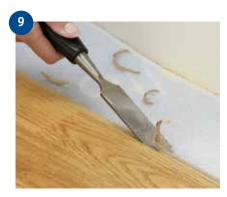
If there is no room to fold down the last board, it can be slide in from the side instead. In order to do this, the tongue of the board in the previous row has to be made level. Use a chisel to shave off the part of the tongue which raises like a bump along the top of the outside edge.
