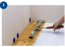
Cut the board where you marked. Angle it into place and tap it in with the pull bar. Place a spacer between the short end and the wall.
