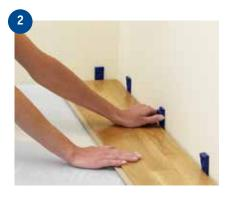
First row. Remember that the floorboards should preferably run along the length of the room. Start in a left-hand corner with the groove side against the wall and work towards the right. The next board is angled down into the short end of the previous board so that it slides into place. Press spacers between the floor and the wall to create an expansion gap of 8-10 mm, after approx. 3 rows is recommended.
