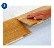
Second plank, first row. Place it gently and tight to the short end of the first one. Fold the panel down in a single action movement. During the fold down, make sure the panels are tight against each other.
