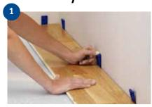
First row. Remember that the floorboards should preferably run along the length of the room. Start in a left-hand corner with the groove side against the wall and work towards the right. If the wall isn't straight, cut lengthwise. Place the tapping block against the short end of the board and tap the boards together with a hammer. Press spacers between the floor and the wall to create an expansion gap of 8-10 mm.
