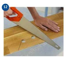
If the long side of the board meets a pipe: Drill a hole with a diameter min. 16 mm greater than the pipe diameter to give an expansion gap around the pipe. Mark with a pencil where to saw. Saw off the bit which will fit behind the pipes, closest to the wall. Cut at an angle as shown in the picture. If the pipes are located along the short side of the floor, cut the board at a 90° angle straight through the holes.
